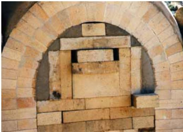
Refractory lining of a furnace arch
