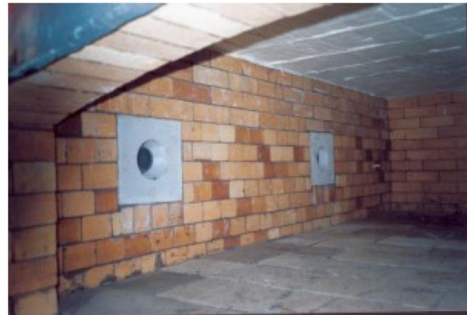
Refractory walls of a furnace interior with burner blocks
